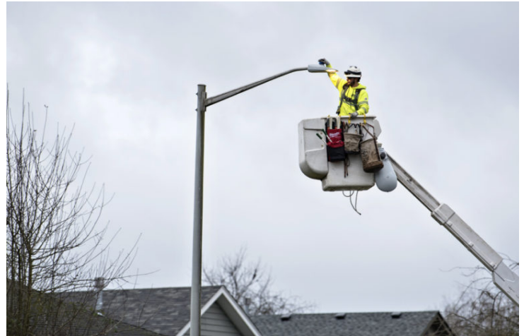
DJ's Electrical lineman Rhett Lindberg of Winlock changes the current high-pressure sodium lights to new LED bulbs in Battle Ground.
