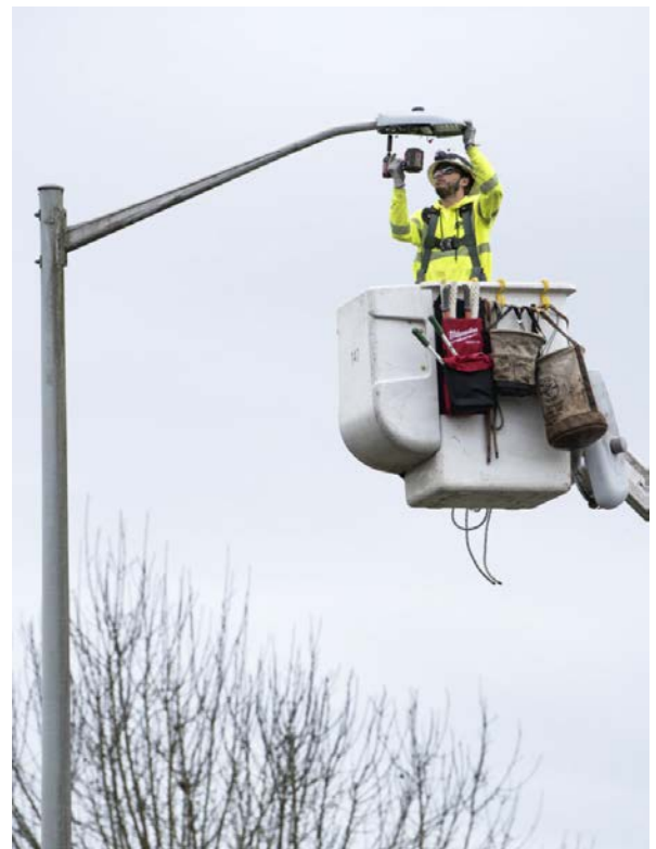
DJ's Electrical lineman Rhett Lindberg of Winlock changes the current high-pressure sodium lights to new LED bulbs in Battle Ground. Alisha Jucevic/The Columbian
