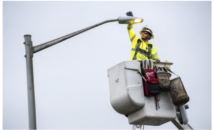
DJ's Electrical lineman Rhett Lindberg of Winlock changes streetlights to LED bulbs in Battle Ground, which teamed up with Ridgefield and Washougal to bid out the replacement work after all three cities received grant money from the Washington State Transportation Improvement Board. Alisha Jucevic/The Columbian
