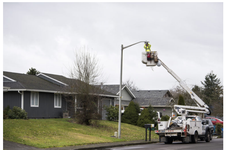
DJ's Electrical lineman Rhett Lindberg of Winlock replaces one of the city's 2,300 high-pressure sodium streetlights to LED bulbs as part of an energy savings initiative in Battle Ground. The project is expected to save the city around $68,000 annually.
