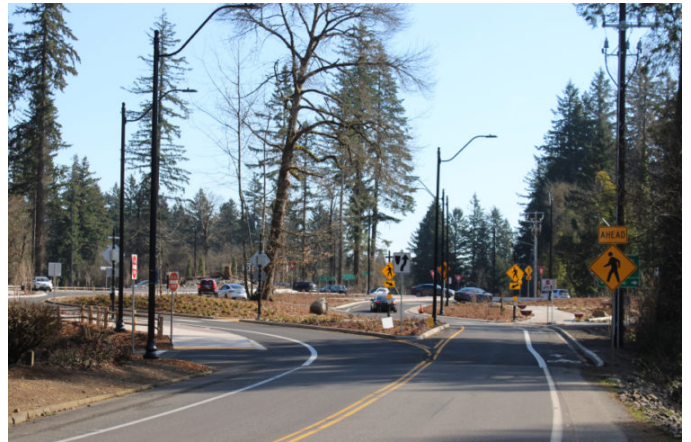
Traffic moves through the newly completed roundabout at Everett Street and Lake Road in Camas on Friday, March 19, 2021.
