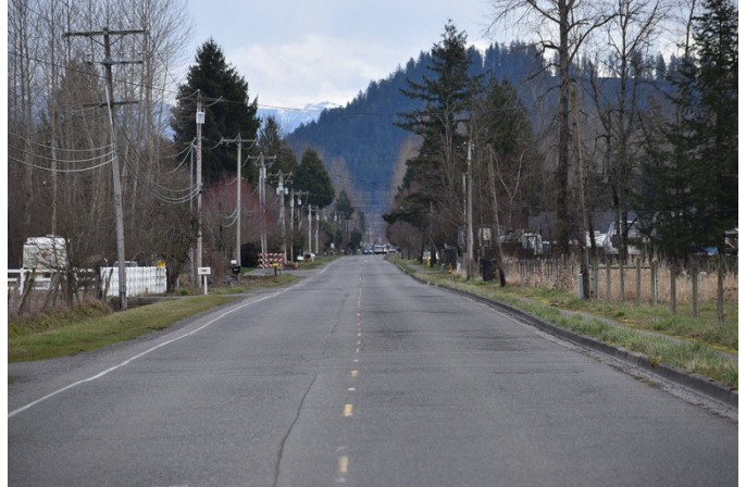
Looking east on March 9 from Mundy Loss Road, the years of wear-and-tear on 112th Street East in Buckley are apparent. The city aims to grind and repave nearly a mile of the road from its intersection at Mundy Loss Road to Highway 165.
