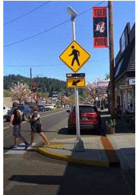
The crossing includes a signal – a flashing light referred to as a Rectangular Rapid Flashing Beacon – that is activated by pedestrians preparing to cross the street. Its bright yellow flashing light serves as a warning to motorists to stop for pedestrians.
