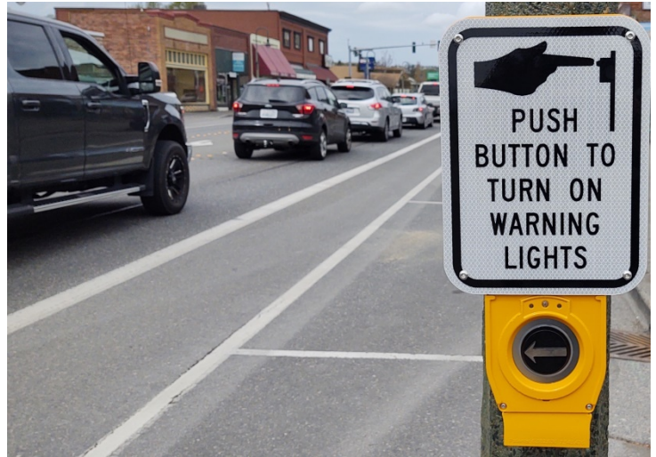
Activator button and instructions with a rectangular rapid flash beacon (RRFB) mounted on a light pole at 1st Avenue and Main Street (April 24, 2020).
