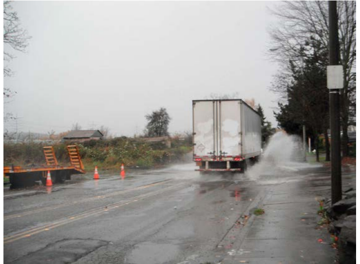
A truck travels through a flooded 76th Avenue South in Kent. A project this year will raise the road so it doesn't flood anymore.
