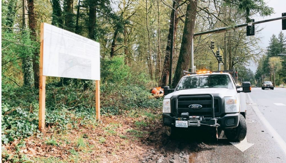
Construction is set to start at the Lake-Everett Road roundabout.
