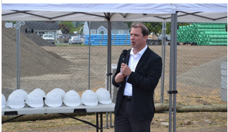
For the West Fir Street Rehabilitation Project, the state’s Transportation Improvement Board funded about $3.1 million of the project. Ashley Probart, Transportation Improvement Board executive director, said the project “clearly is a high priority for the TIB.” The board met in Sequim on May 16-17, as well.
