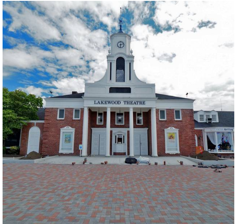
Decorative pavers enhance the pedestrian-friendly Colonial Plaza in Lakewood. City of Lakewood
