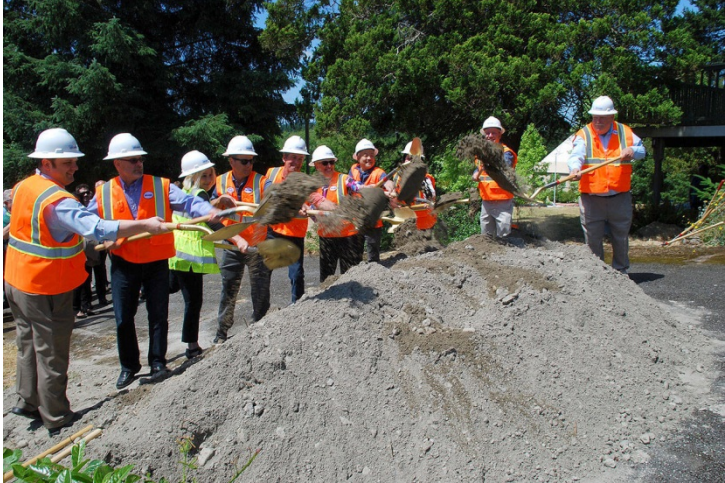
Port Orchard city officials and legislators, with ceremonial shovels in hand, turn dirt to signal the start of construction at the site of the Tremont Street project in July 2017. (Bob Smith | Kitsap News Group 2017)
