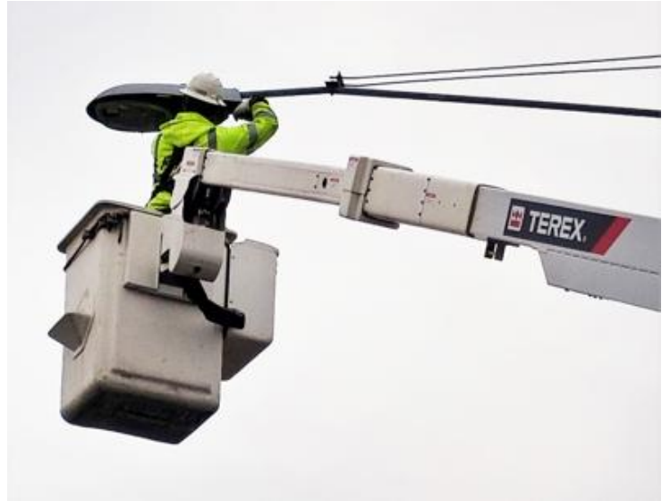
A PacifiCorp lineman replaces mercury vapor lighting with new LED lighting in Sunnyside. City of Sunnyside
