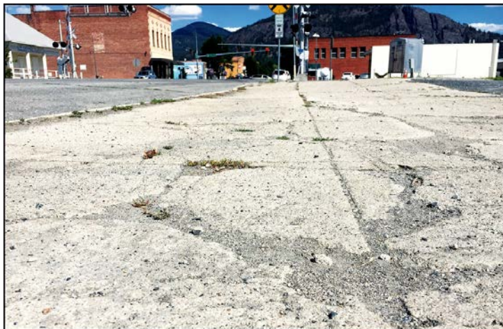
Sidewalk construction will begin around some of Chewelah's busiest areas. (Brandon Hansen photo)
