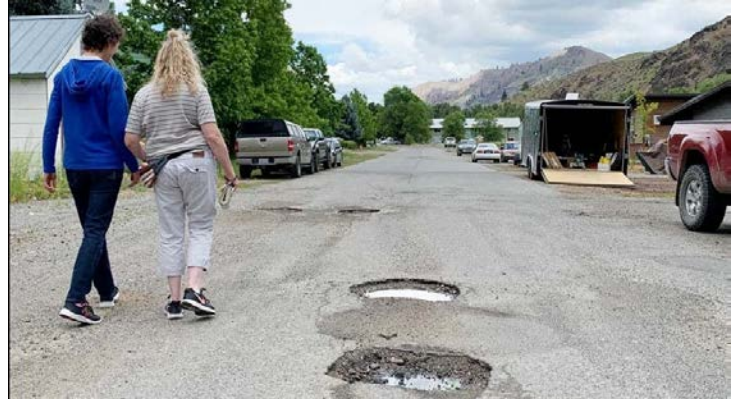
Audrey Ludeman, left, and Marilyn Marr of Twisp dodge potholes Thursday (June 27) while walking north on Canyon Street in Twisp. Construction work, including water-line replacement, sewer repairs and a new sidewalk, started this week.
