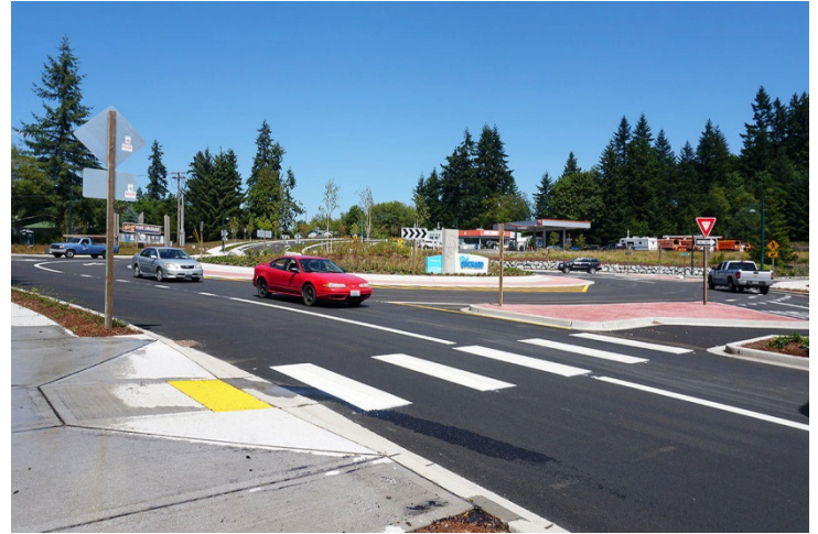
Tremont Street reopened to traffic at the completion of the 25-month construction project on July 29. (Bob Smith | Kitsap Daily News)
