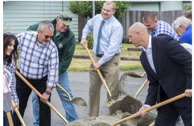
Officials from Centralia and Lewis County, including Commissioner Bobby Jackson and Gary Stamper, second and third from left, participate in the ceremonial groundbreaking of the Borst Avenue project on Thursday.
