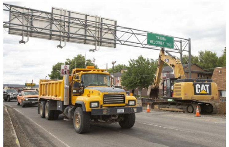
Construction crews work on North First Street on Wednesday in Yakima.
