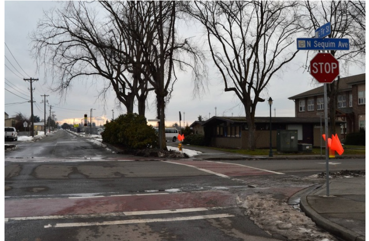
North Sequim Avenue closes at West Fir Street temporarily from 5 p.m.-midnight on Monday, May 13, and Tuesday, May 14, for construction as the start of the West Fir Street Rehabilitation Project. Detours will be in place. Sequim Gazette file photo by Matthew Nash
