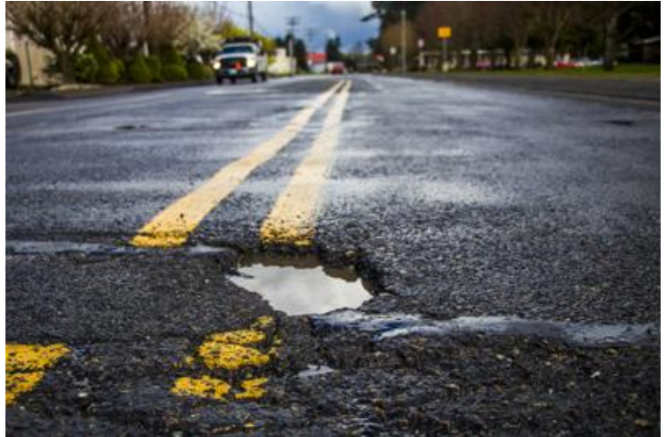
A pot hole is seen in the center of Borst Avenue as vehicles make their way down the road in April in Centralia.
