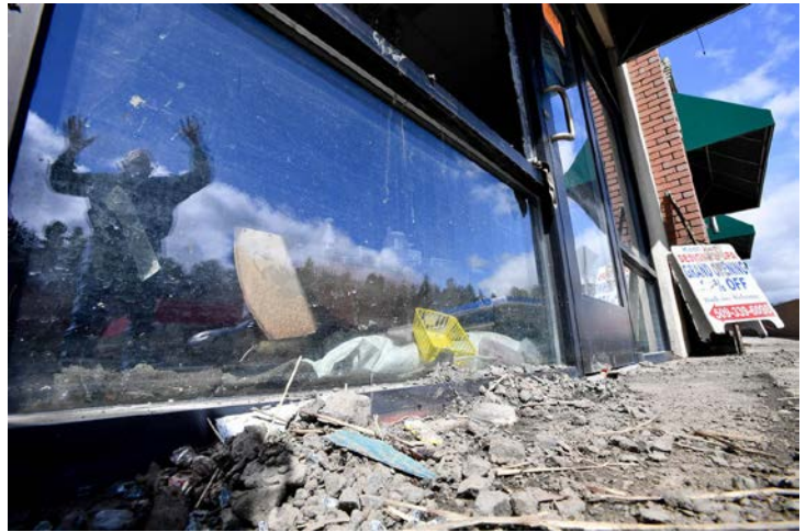
Parley Pearce, of Walla Walla, is reflected in the window of a building he owns at 745 N. Grand Ave. in Pullman on Wednesday, April 10, 2019. He gestures at one of his tenant's businesses, a nail salon that was damaged by flooding the previous night. "These are really hard-working people," Pearce said. "I hate to see this happen to them." (Tyler Tjomsland / The Spokesman-Review)
