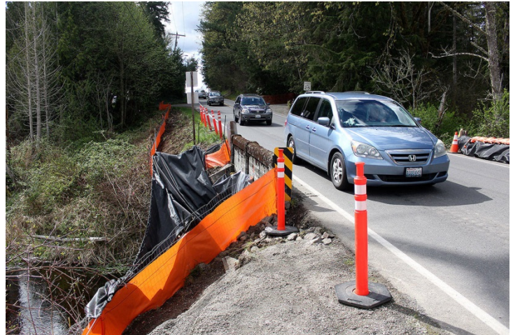
A pedestrian bridge is being installed on Black Diamond's Rock Creek Bridge's south side, which will allow foot traffic to cross the bridge more safely. Some concerns were raised about the project being exempt from the state's SEPA process — maybe especially because Rock Creek is a salmon-bearing bridge — but erosion control and debris mitigation measures have been set up.
