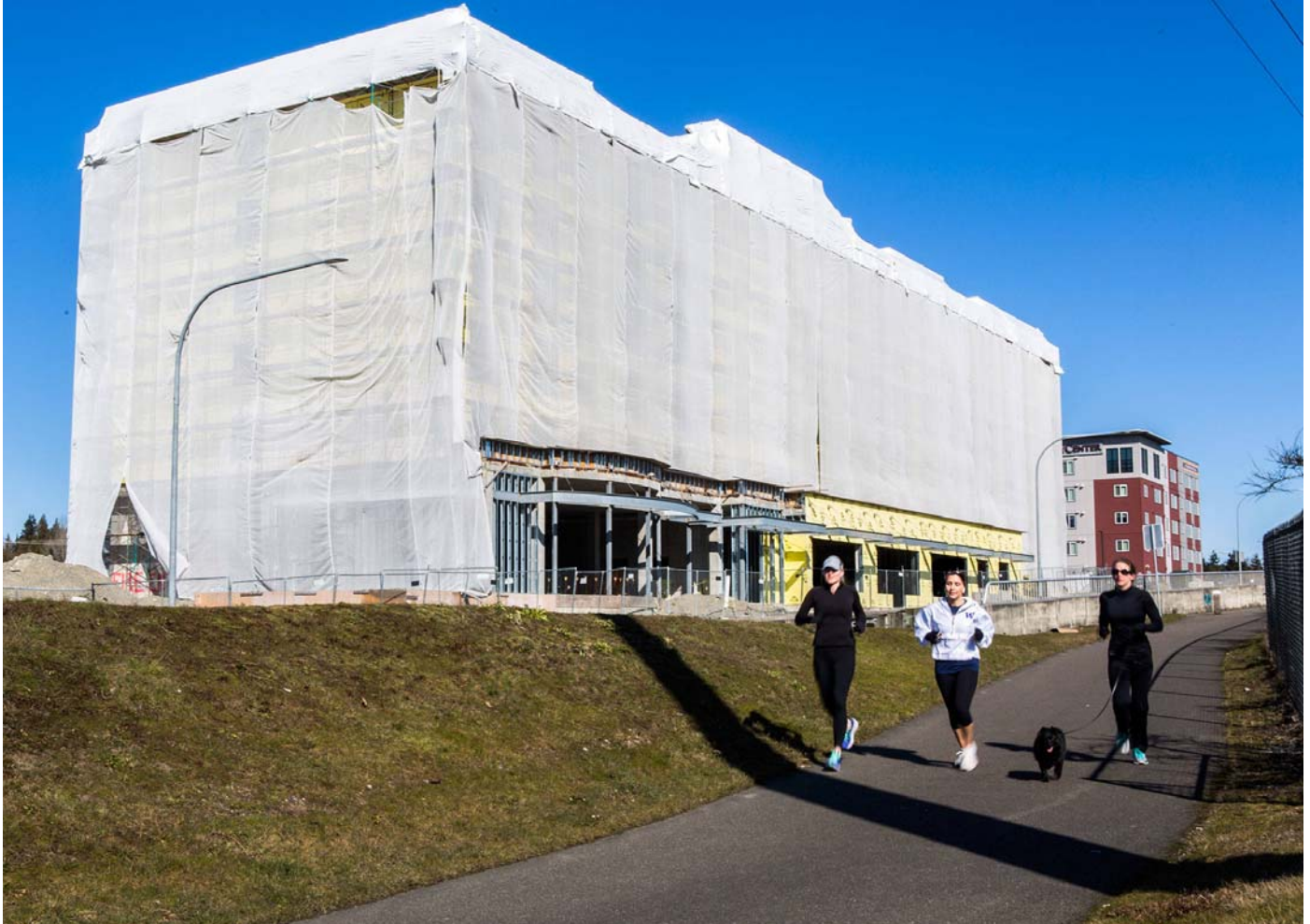
Joggers on the Interurban Trail run past a Hilton Garden Inn under construction on Friday, March 1, 2019 in Lynnwood, Wash. (Olivia Vanni / The Herald)
