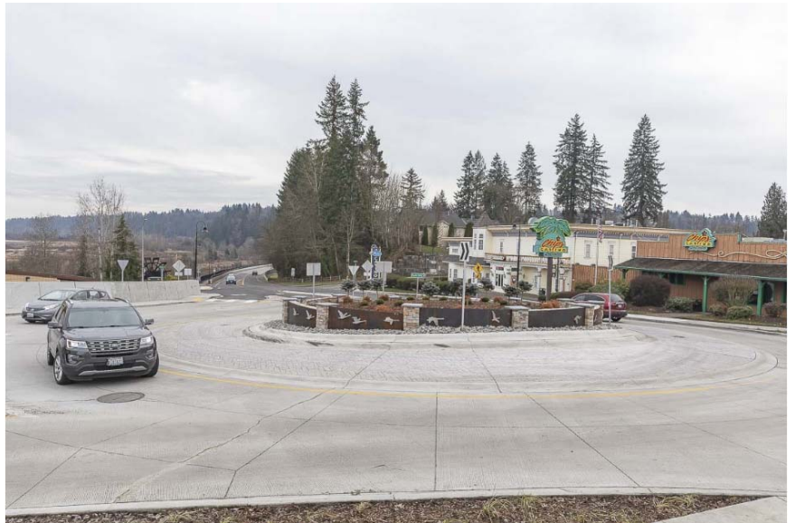
The roundabout construction project was completed in December 7, 2018.
