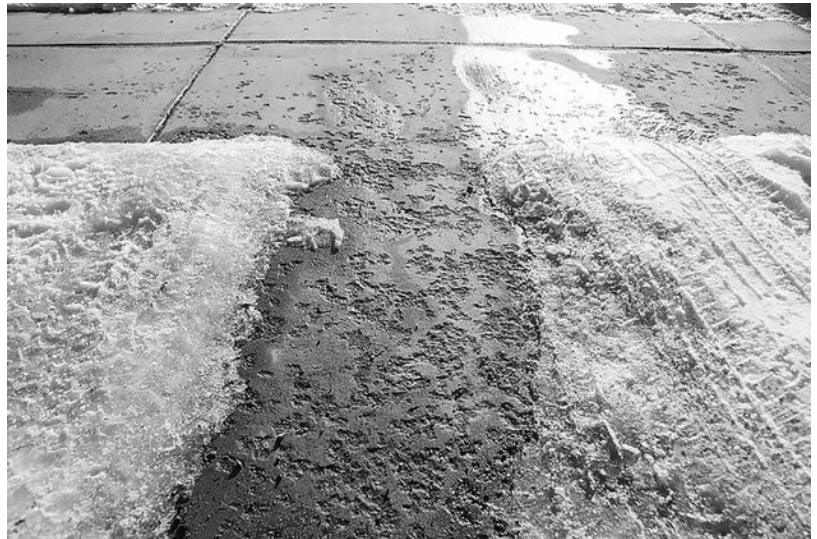
A sidewalk on Main Street exhibits "spalling," one of the problems under contention with the new walkways. - Jacob Wagner photo
