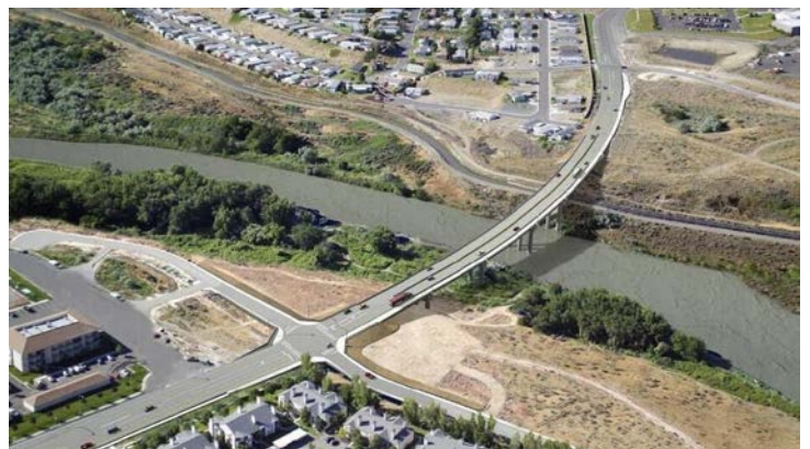
Richland's new bridge will carry Duportail Street across the Yakima River when it opens in 2020. Apollo Construction, the contractor, is building the bridge's easternmost bridge support, shown in the forefront of this rendering. Image courtesy city of Richland
