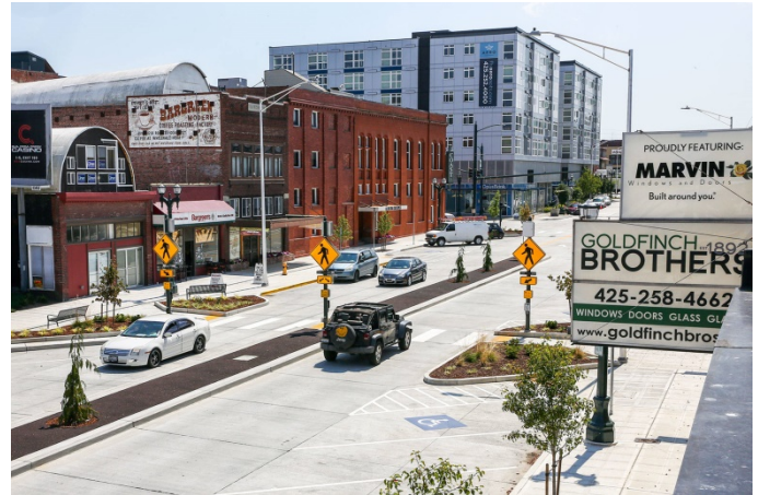
The Rucker Renewal project wrapped up in July 2020 for through traffic, but change orders over the yearlong construction added almost $2 million to the original $9.5 million budget. (Kevin Clark / Herald file)
